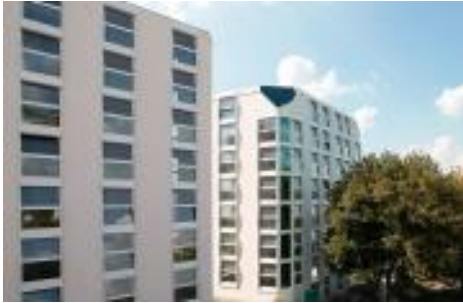
Fig. 7.5: Exterior view of the residential building Rautistrasse, Zurich
